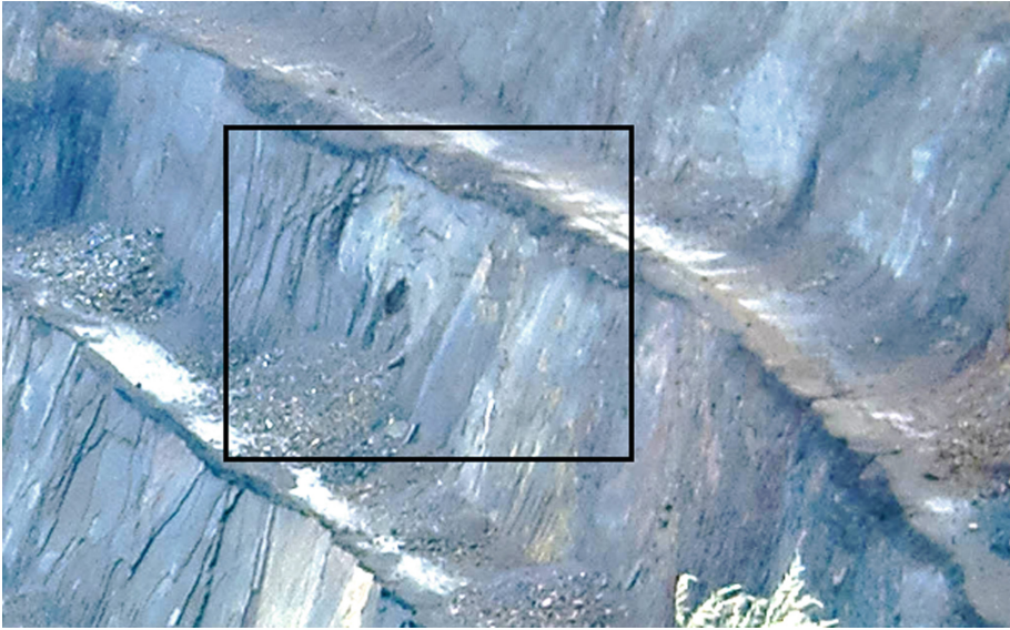
Fig. 3. Sidewall spalling in the face of the pit bench, photo taken from the south in February 2011
