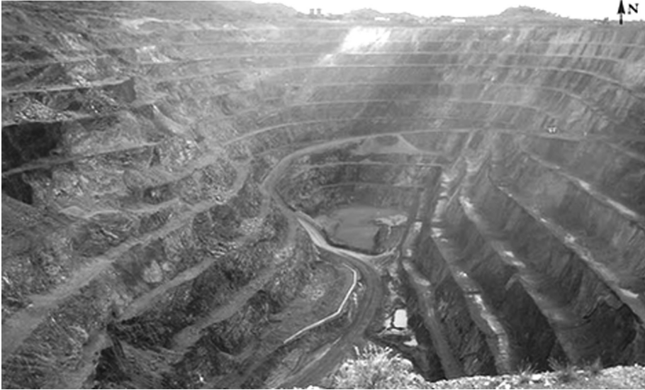
Fig. 1. View of Handlebar Hill open pit, photo taken from the south in February 2011
